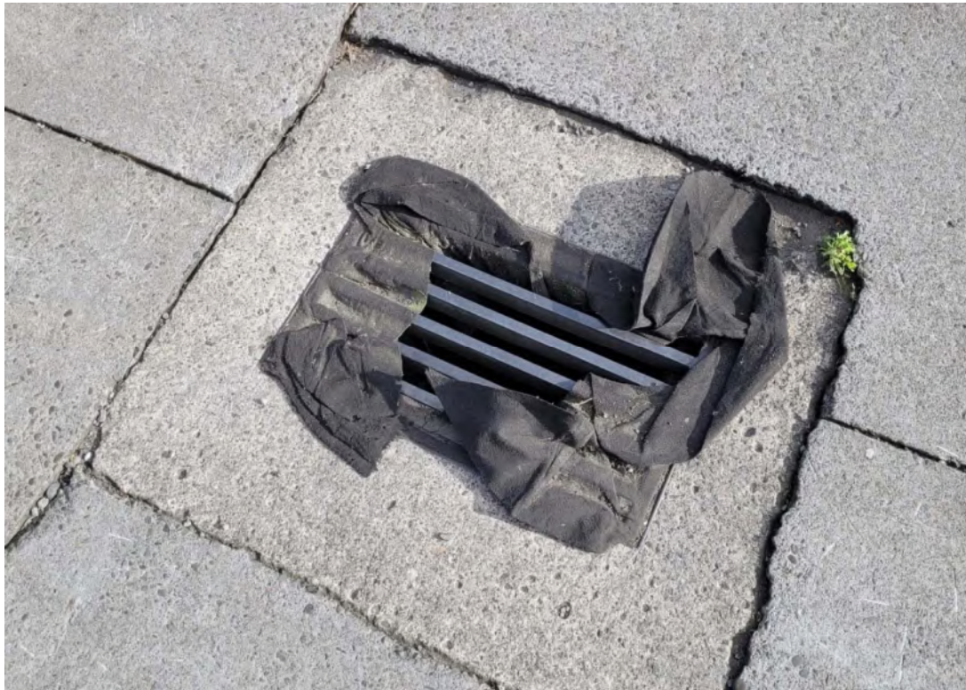
Photo 4 Drain sock in place, May 2022
