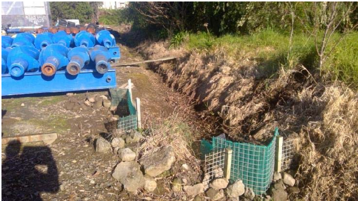
Photo 19 Sediment controls on Tasman Tools' perimeter drain, September 2020
