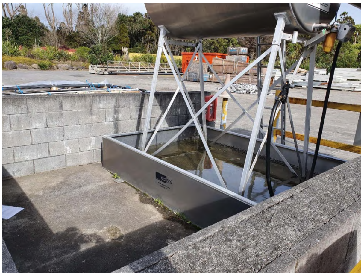
Photo 13 Hazardous chemical storage and bunding, July 2020
