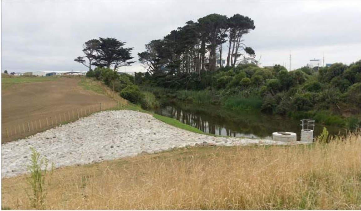
Photo 4 Southern stormwater pond following upgrade (surrounded by native riparian plantings)
