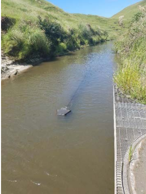
Photo 2 Tangahoe River intake structure
