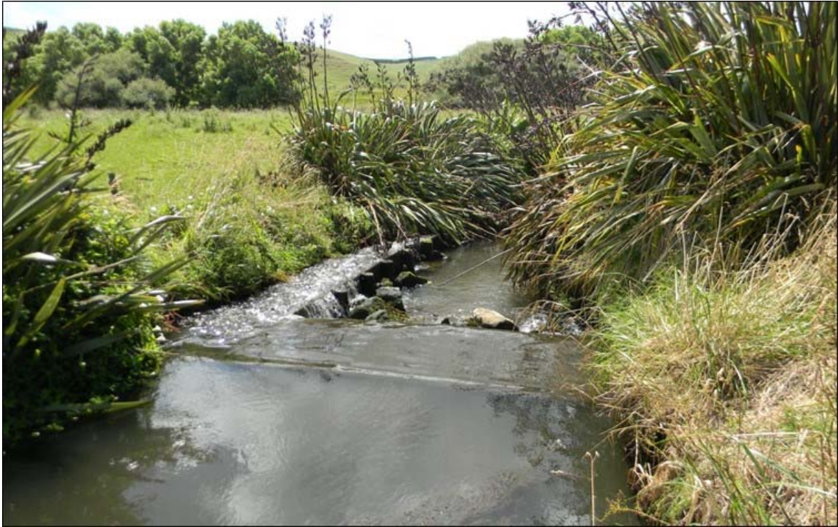
Photo 3 The weir and fish pass on the Tawhiti Stream
