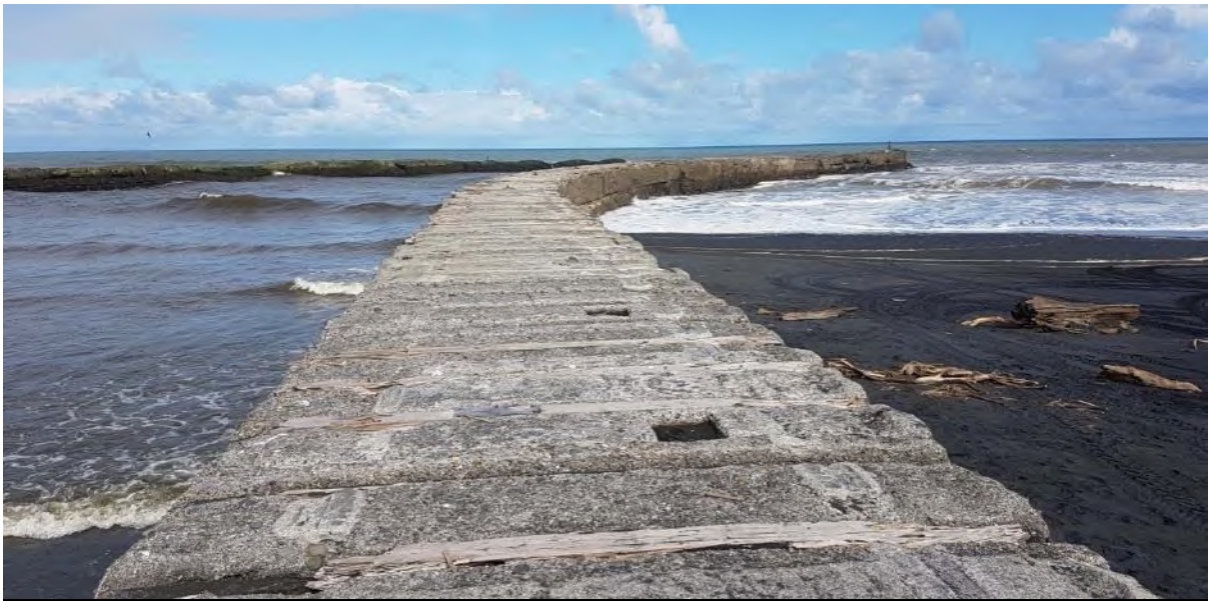
Photo 5 Patea groynes (April 2017)
