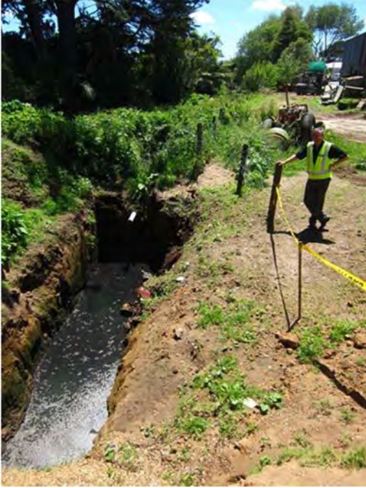
Photo 1 The third settling pond
