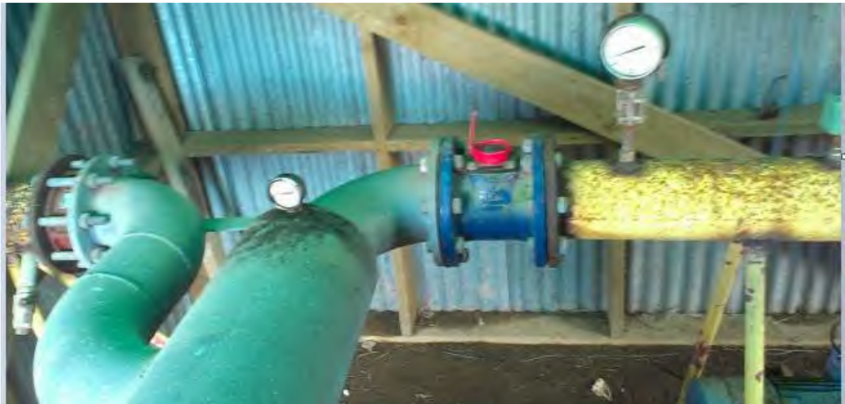
Photo 5 Example of a poor flow meter installation
