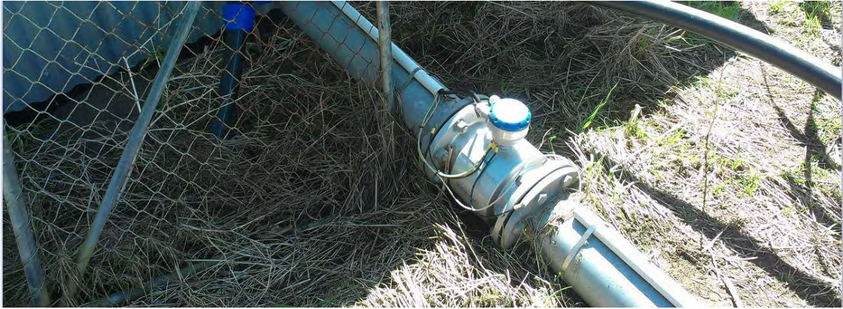
Photo 4 Example of a good flowmeter installation
