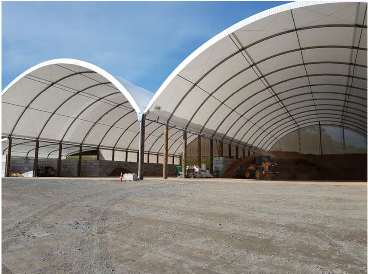
Figure 2 Osflo facility during construction both sides of the depot visible
