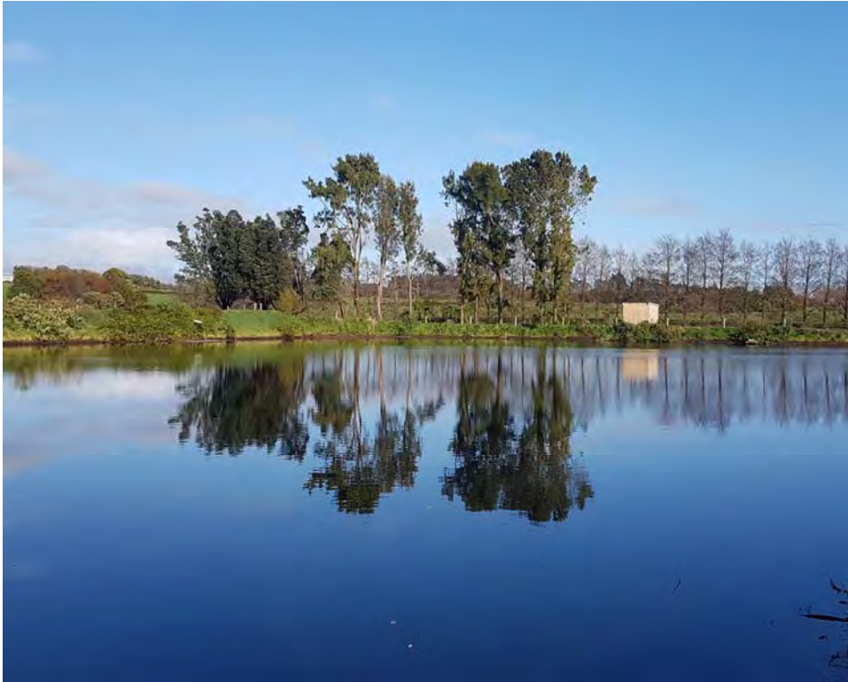
Figure 11 New pump shed recently built on the final aerobic pond for spray irrigating treated piggery effluent to land
