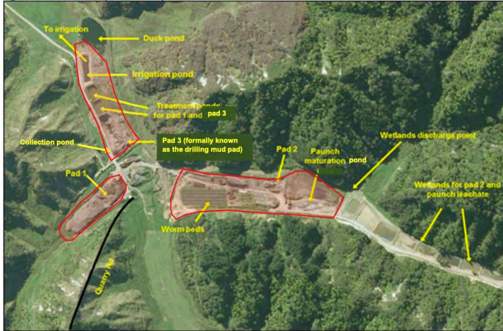
Figure 1: Identification of operational components
