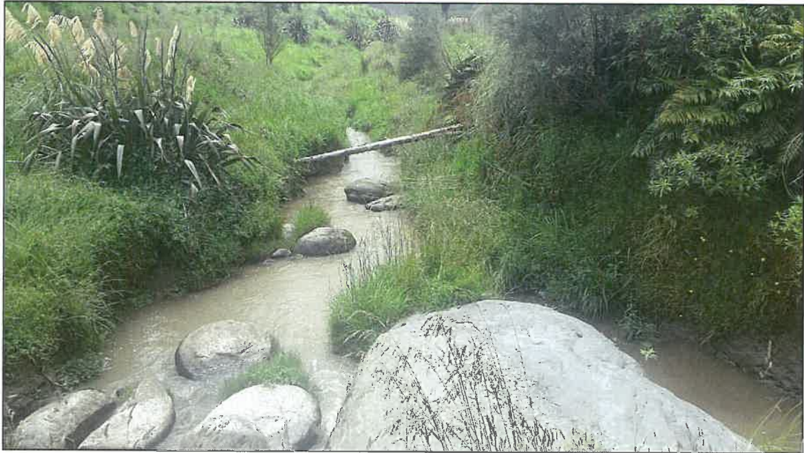
Photo 2 Water clarity at site 1 (top) and at the culvert near the composting pads (bottom). Photos taken about 30 minutes apart.
