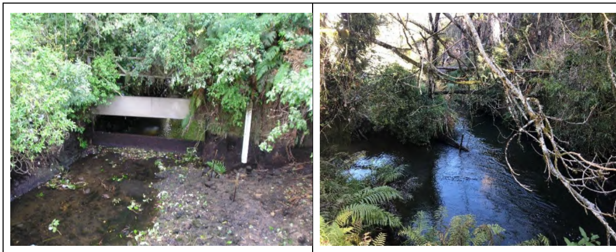
Figure 2.12: Photos of the tail race immediately downstream of the Power Station (left) and where the tail race joins the Makara River (right), with the Makara River coming from the right of the photo. Source: Trustpower
