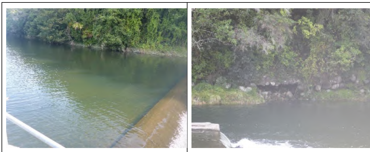
Figure 2.6: Photos of the Manganui River near the Manganui Weir showing the trapping of sediment upstream of the weir (left) and the bank material (right). Note the difference in bank height between upstream and downstream. Source: Author's photos
