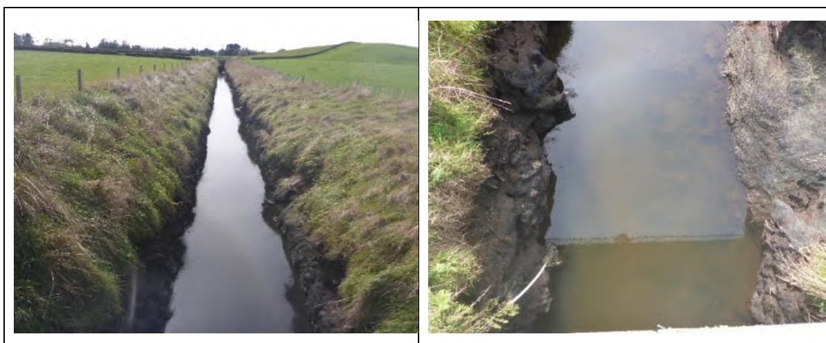
Figure 2.9: Photos of the Motukawa Race diverting water from the Manganui River to Lake Ratapiko. Note the pieces of eroded bank still on the bed in the photo on the right. Source: Author's photos
