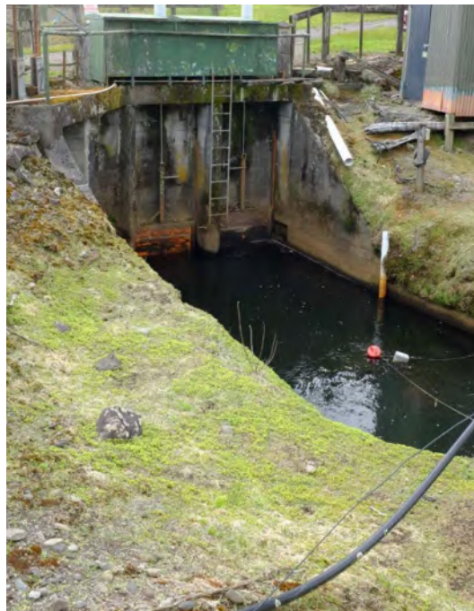
Figure 4.15. Sluice gate channel, November 2018. Motukawa HEPS sluice gates.
