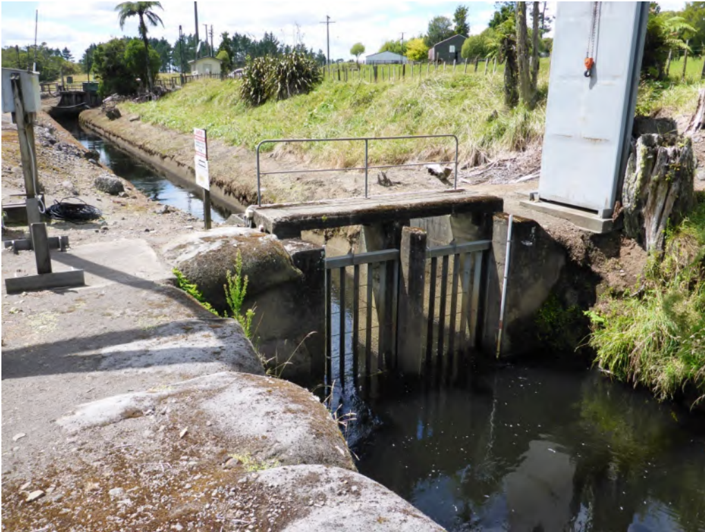
Figure 1.4. Motukawa HEPS intake structure on the Manganui River, February 2021.
