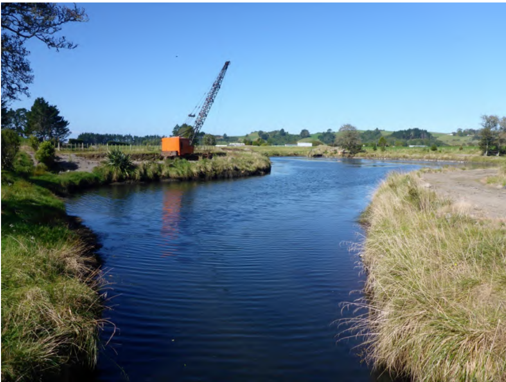
Figure 1.5. Settling pond, April 2021.
