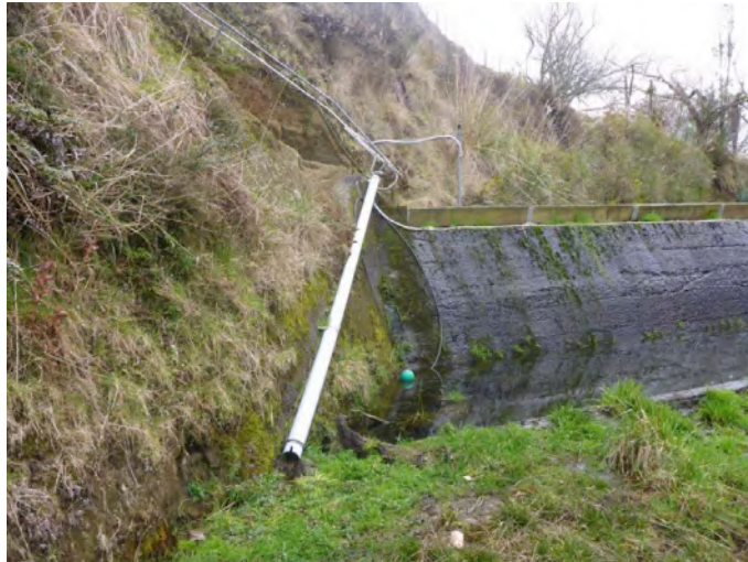
Figure 4.18. Elver pass at Lake Ratapiko spillway, August 2019 (pass not operating at the time).
