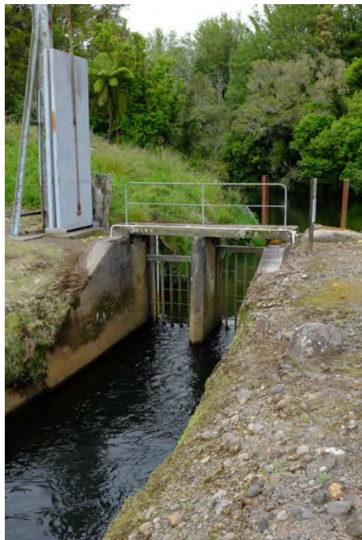
Figure 4.14. Motukawa HEPS trash rack on the Manganui River intake, November 2018.
