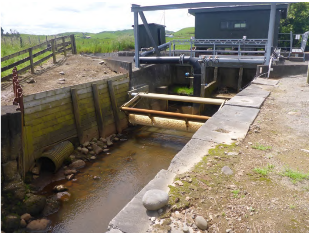
Figure 1.7. Mangaotea Stream pump structure, November 2018.
