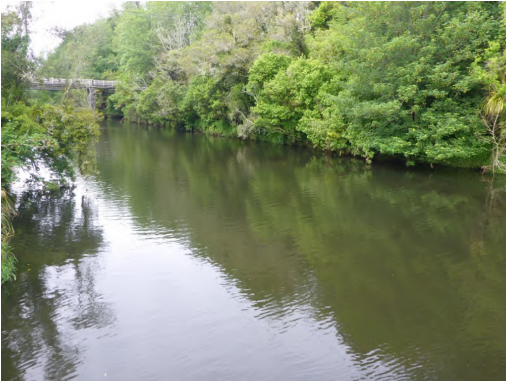
Figure 1.2. Manganui River upstream of the Motukawa HEPS intake structure and weir, November 2018. Tariki Road South bridge visible in background.
