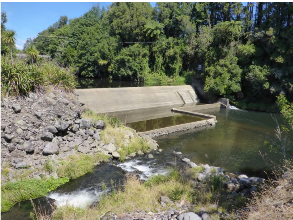
Figure 1.3. Motukawa HEPS intake weir and fish passes (left foreground and right background) on the Manganui River, February 2020.
