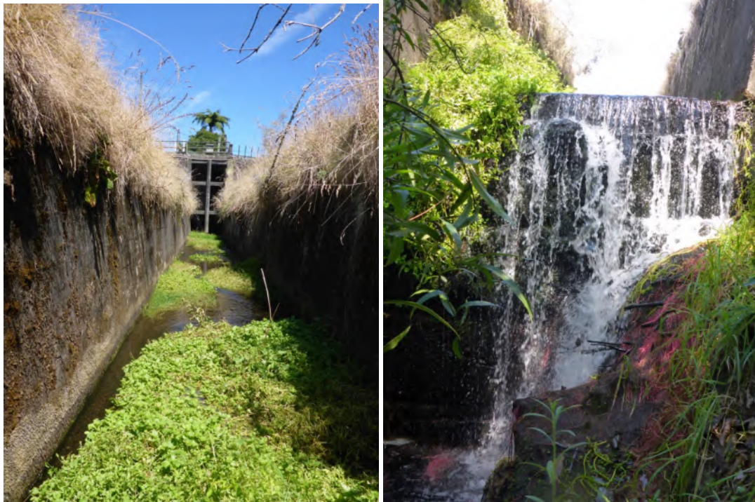
Figure 4.16. Sluice gate channel, February 2020. Left: Looking up channel towards sluice gate. Right: Downstream end of the channel at the Manganui River.
