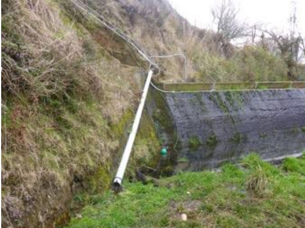
Figure 8: Ratapiko Dam Spillway Elver Pass
