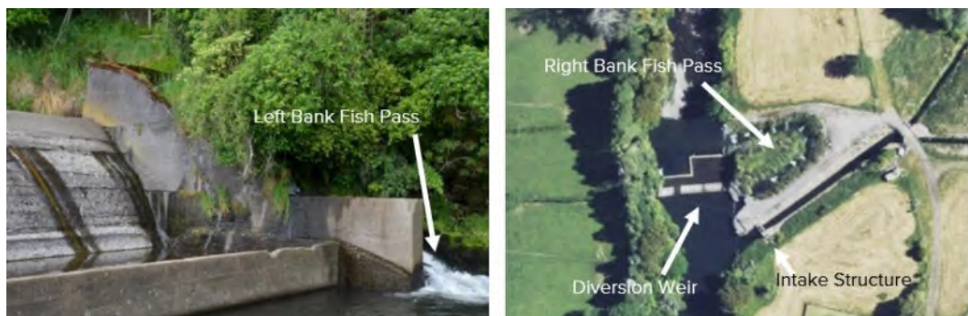
Figure 5: Motukawa Race Intake Components
