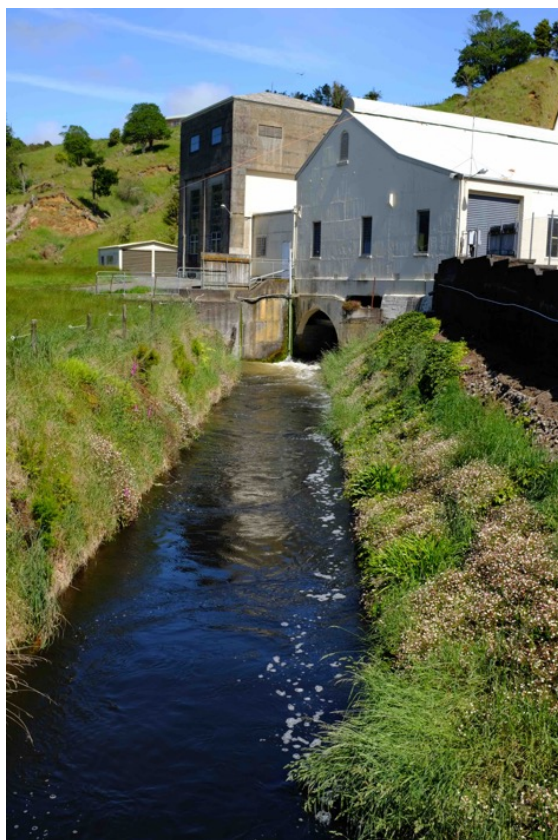
Figure 1.9. Mangorei Power Station with tailrace canal in the foreground.
