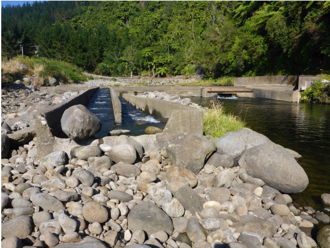
Figure 1.2. Mangorei HEPS low-head weir and fish pass on the Waiwhakaiho River.
