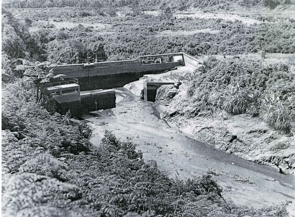
Figure 4.7. NPDC dam in the lower Mangamahoe Stream c.1950. The downstream dam was built in 1914 but washed out, and was replaced in 1917-1918 by the upstream dam. (Photo J. A. Austin, PHO2002-826, Puke Ariki Collection).
