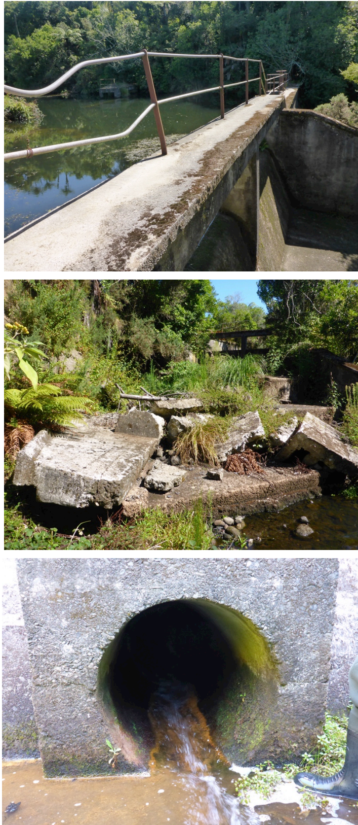
Figure 3.18. NPDC Dam in lower Mangamahoe Stream, February 2020.
