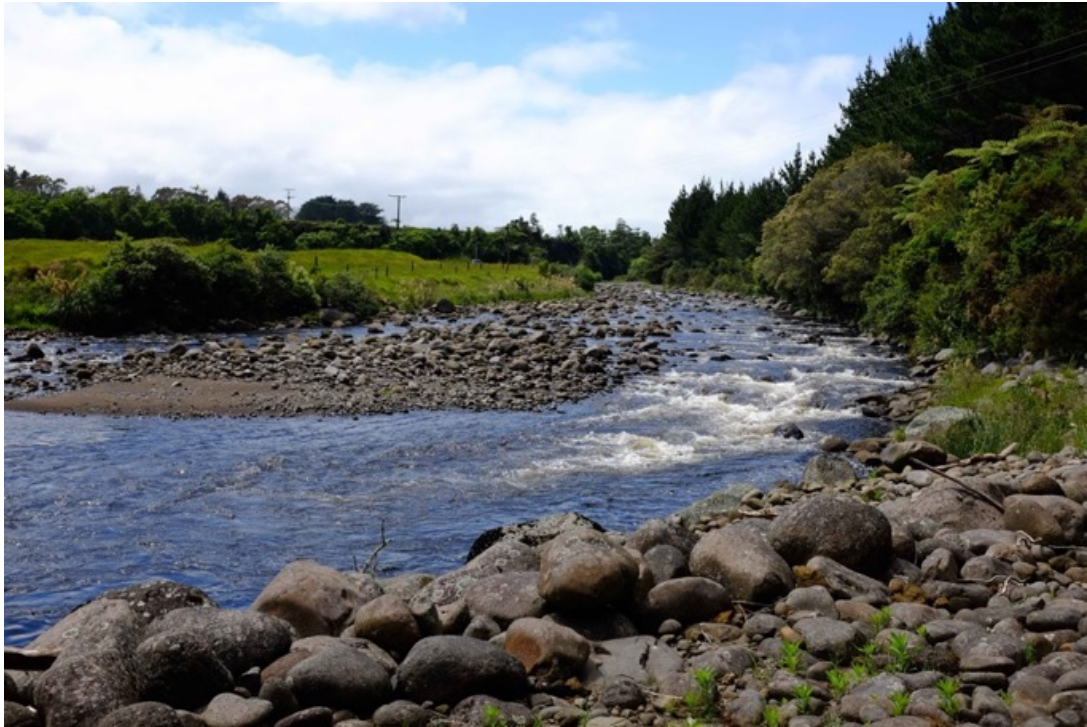
Figure 1.4. Waiwhakaiho River upstream of the Mangorei HEPS intake structure.
