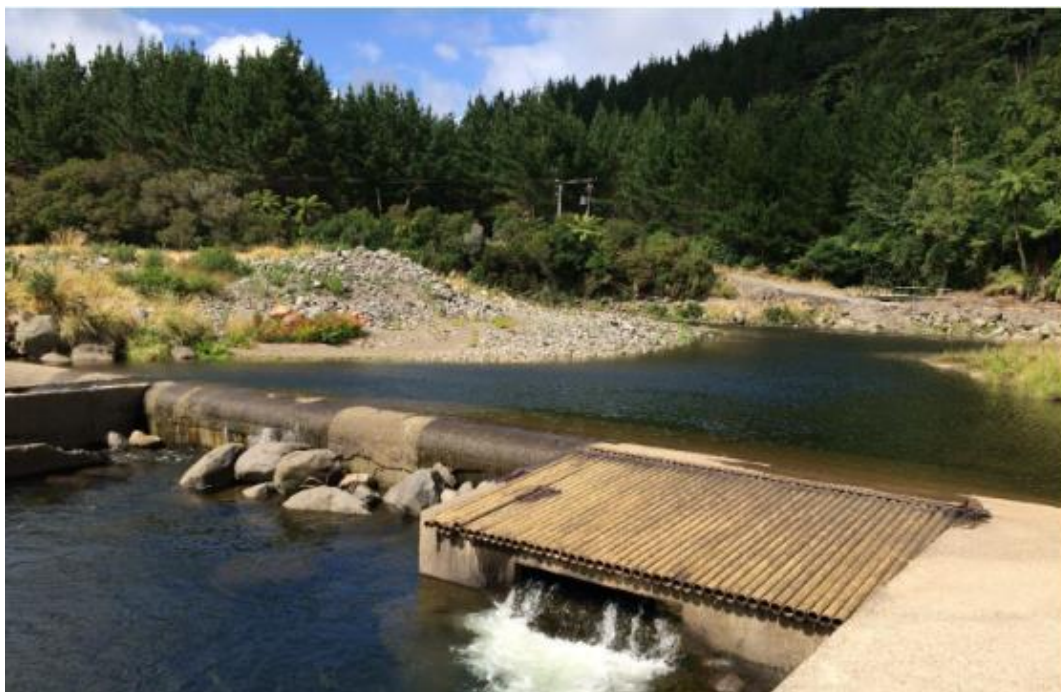
Figure 3.2 Intake weir on Waiwhakaiho River looking upstream (photo credit: Riley 2019)
