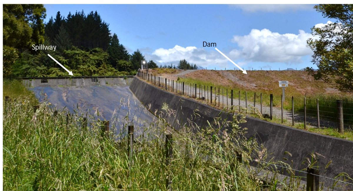
Figure 3.8 Mangamahoe Dam (on right in background) and spillway (on left in foreground)
