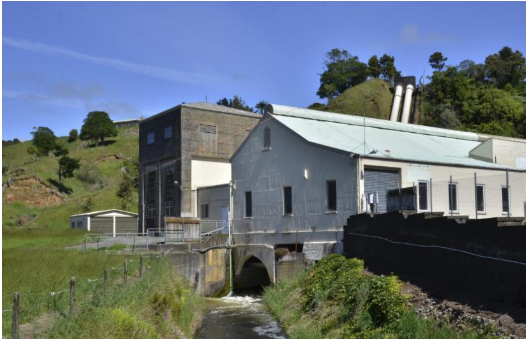
Figure 3.15 Mangorei Power Station. Twin penstocks visible in the background at top right and tailrace in the mid-foreground
