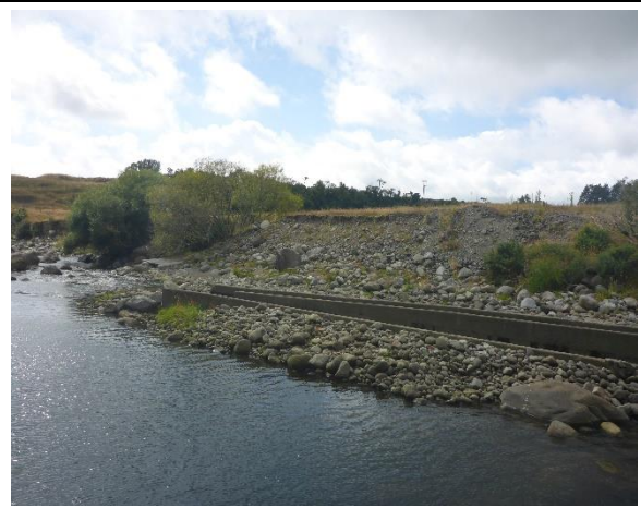
Large boulders downstream of the weir on the Waiwhakaiho River. Banks of boulders and gravels held in a loose sand matrix.
