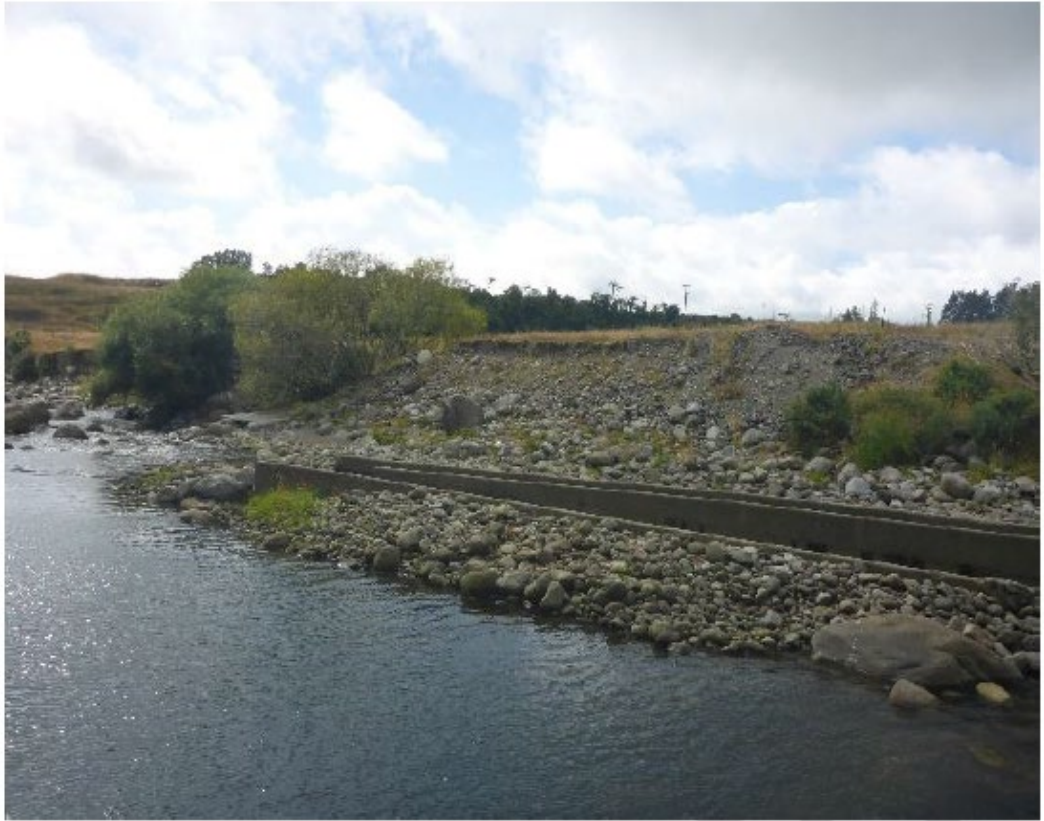
Figure 7: True Right Bank of the Waiwhakaiho River where Boulders and Debris are Placed Following Removal
