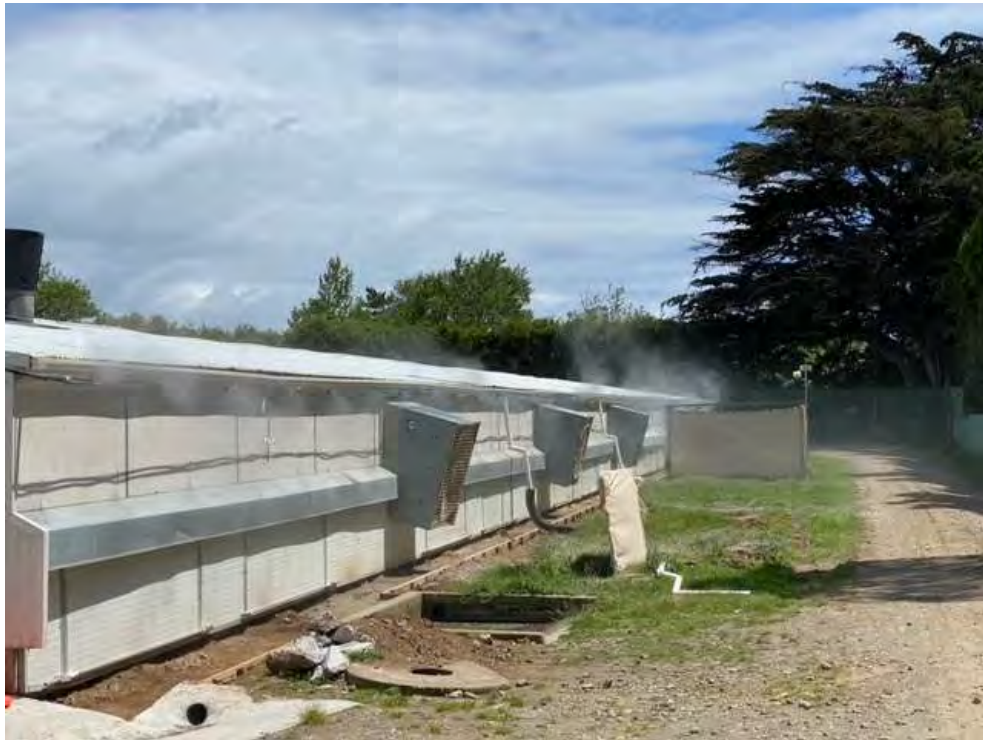
Photo 8 Sidewall misters and fan misters in operation
