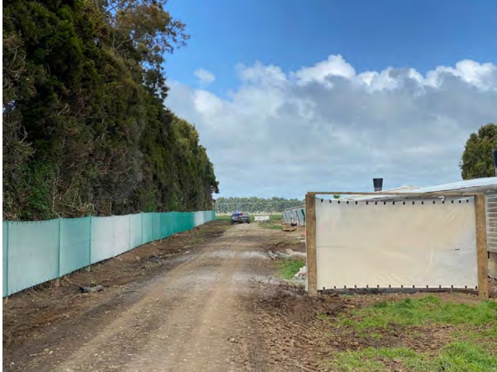
Photo 9 Dust emissions and controls (21 September 2021)
