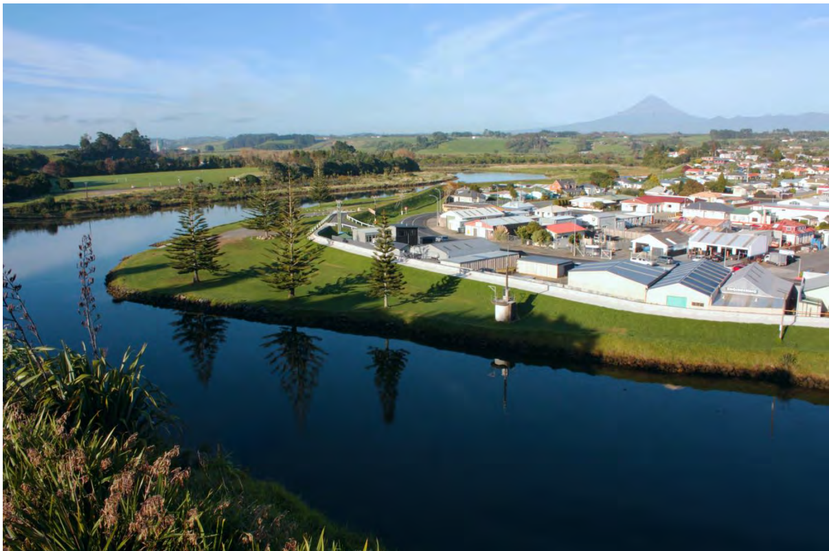
Image: Waitara River stopbank West Quay from Manukorihi
