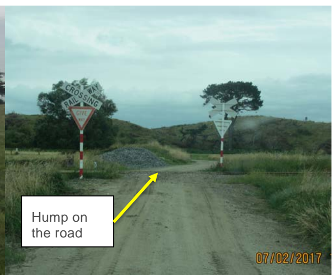
Figure 2-6: Hump on the Road at the Level Crossing
