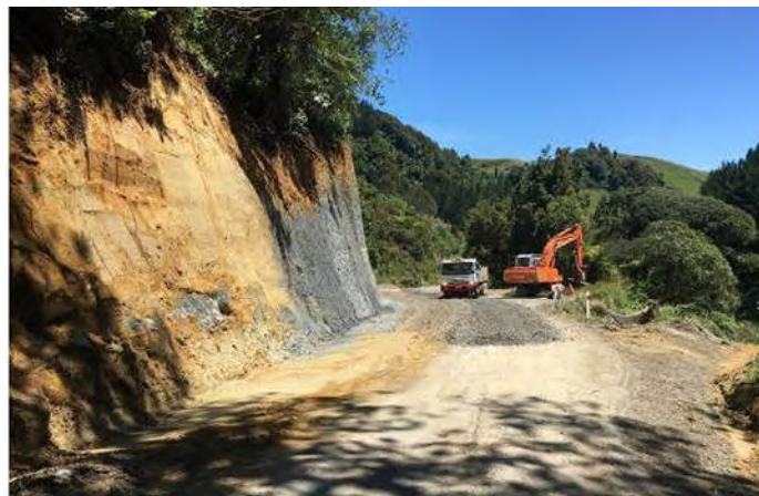
Mangaoapa Road – bank trimming and road strengthening for logging operations.
