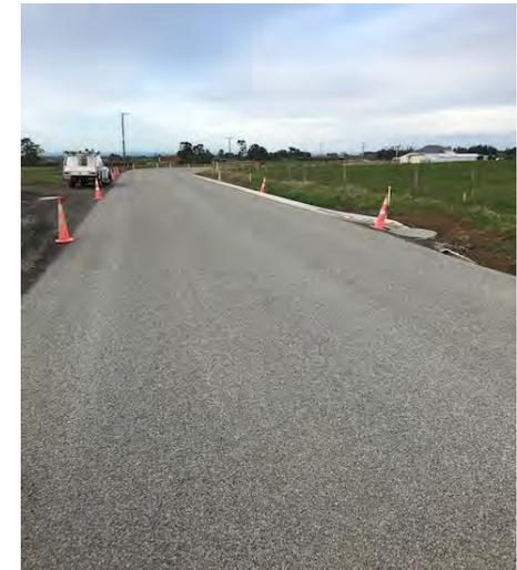
Later in the year SDC were given approval to commence on the upgrade of the Plateau carpark on Pembroke Road. This involved the construction of a concrete footpath around the perimeter of the carpark, placing rocks to control surface water run-off and sealing of the carpark surface. Unfortunately, the cold weather beat us, resulting in the carpark not being sealed. This will be undertaken later this year, when weather conditions are more suitable for sealing.
