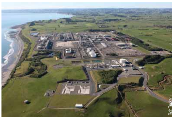
Methanex methanol plant and the Pohokura production station in foreground, Motunui.
