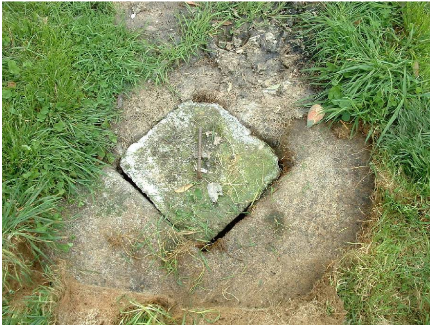
Photo 9 Typically constructed offal hole with concrete cap and lid
