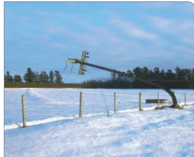
Power poles brought down by the weight of snow during the June 2006 Canterbury snowstorm. The snowstorm left thousands of people in South Canterbury without power for up to 4 weeks. Electricity Ashburton.
