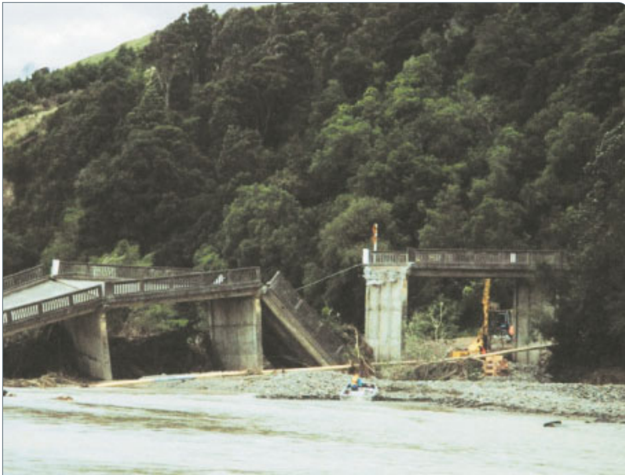
The Saddle Road bridge over the Pohangina Bridge in the Manawatu after the February 2004 storm. The bridge carried the main gas transmission line between the Manawatu and Hawke's Bay and its loss affected food processing industries in Hawke's Bay. Westmoreland School.
