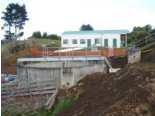
Photos 6 and 7 Pump base at rear of old clarifier, May 2009
