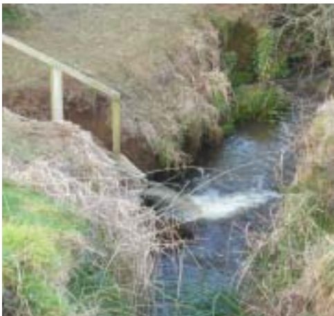
Photo 5 New access to outfall, June 2009
