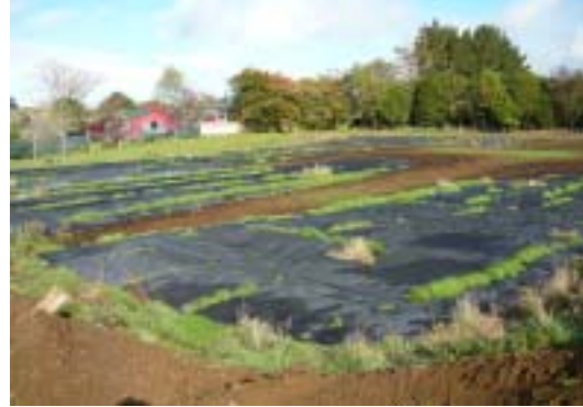
Photos 1 and 2 Water treatment plant sludge and geotextile WWTP sludge bags, May 2009
