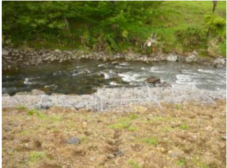
Photo 3 Relocated river riprap outfall
