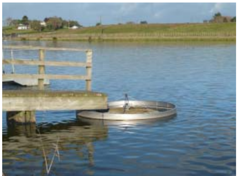
Photo 2 Primary pond outlet access jetty
