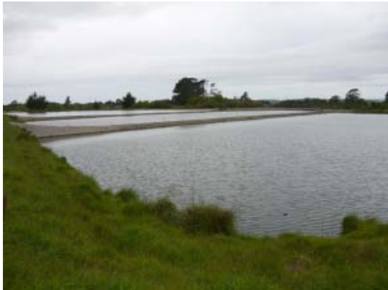
Photo 5 Division of second oxidation pond into three cells, November 2008
