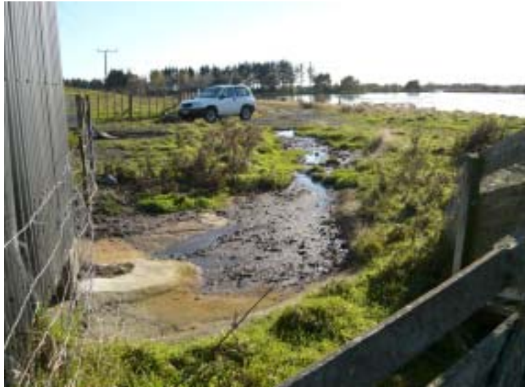
Photo 4 Overflow from step-screen area to primary pond, May 2009
