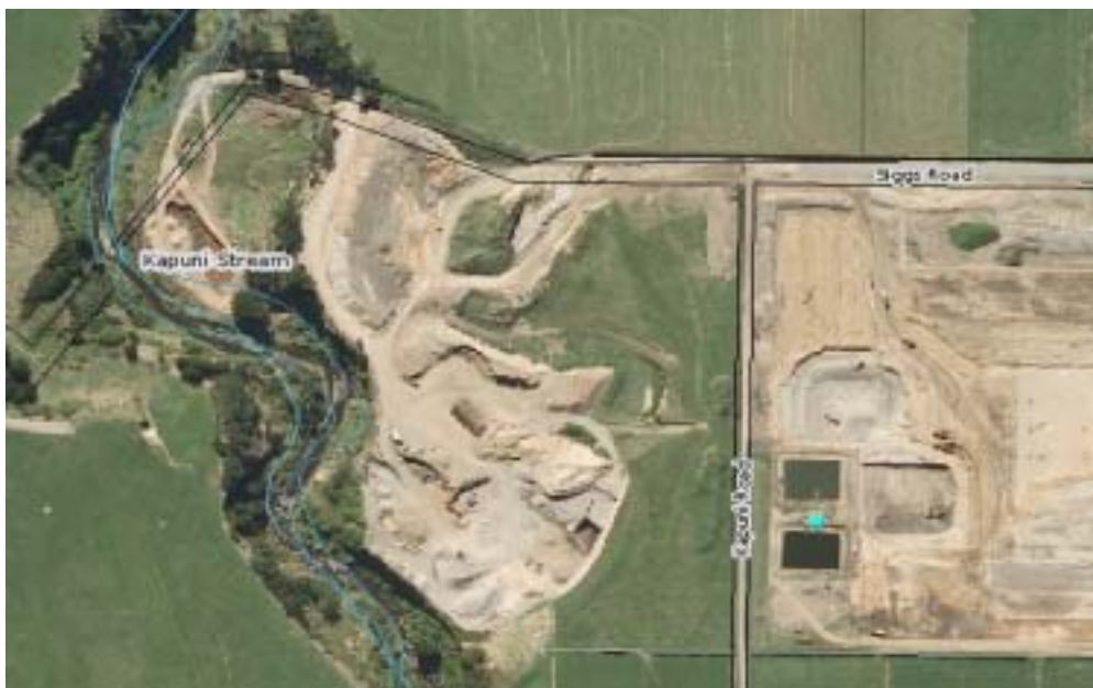
Figure 2 The development of the Kupe site adjacent to quarry
