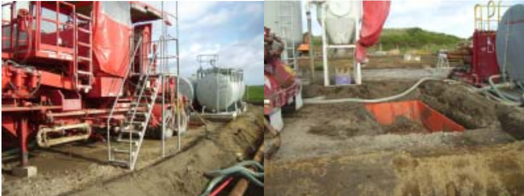
Photo 4 Bunding/containment around the Halliburton cement truck
