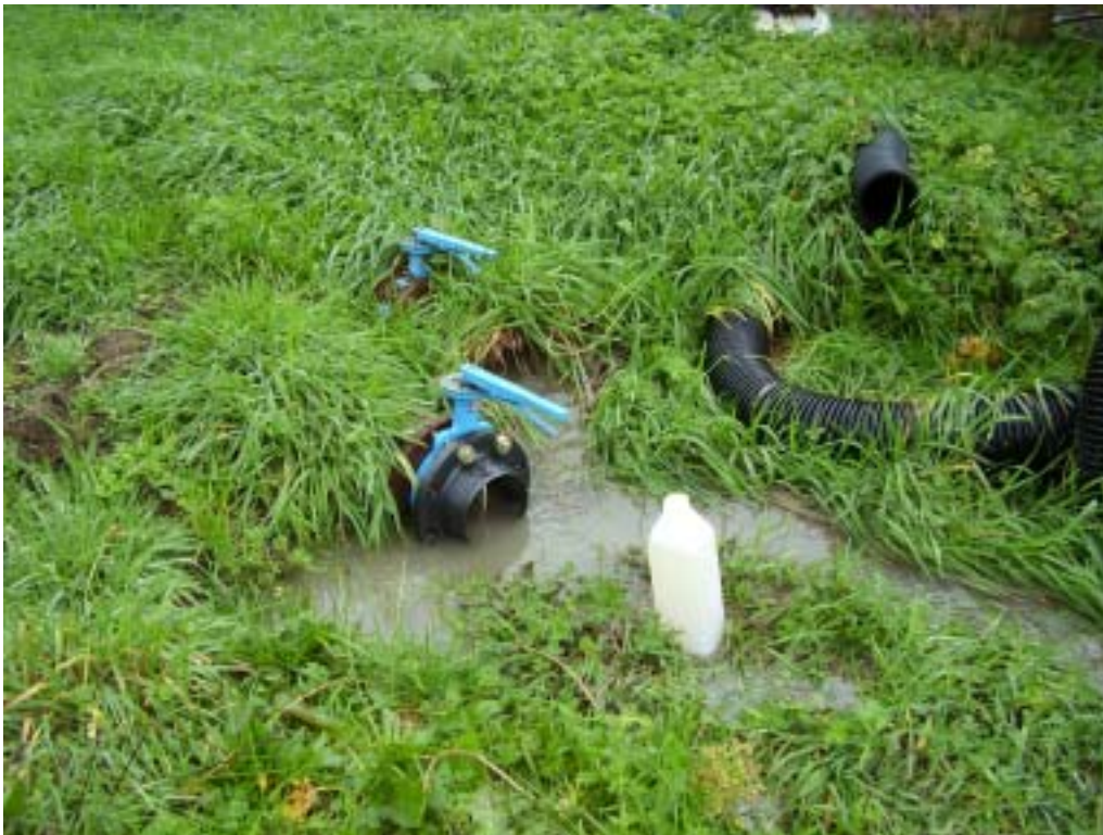
Photo 1 Water sample collected at the discharge point from the skimmer pits
