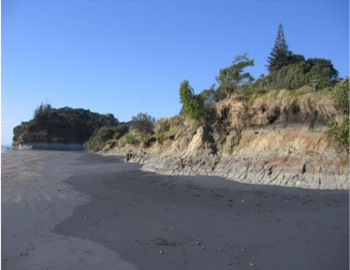
Photograph 1 Erosion on Wai-iti foreshore prior to construction of the rock rip rap seawall
