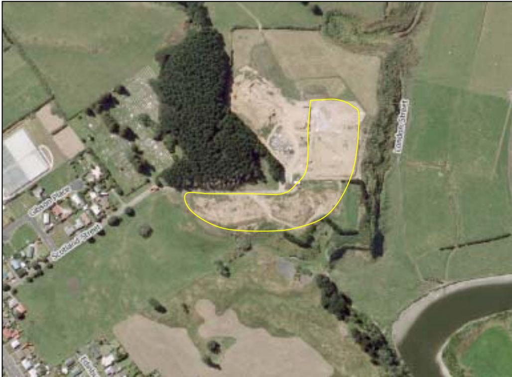
Figure 7 Aerial view of the landfill at Patea
