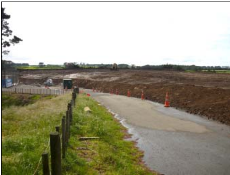
Photograph 1 Patea Landfill during early stages of capping works, 24 October 2009
