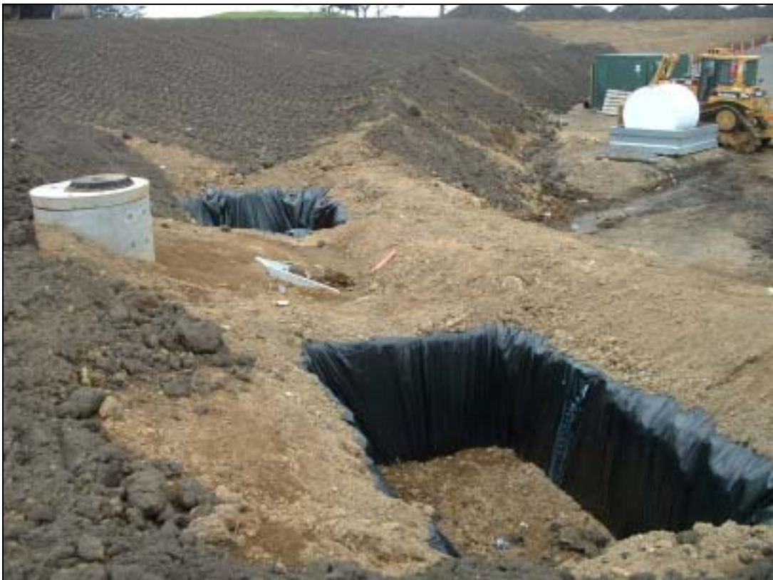
Photograph 2 Plastic lined silt traps on north side of cap, 4 November 2009
