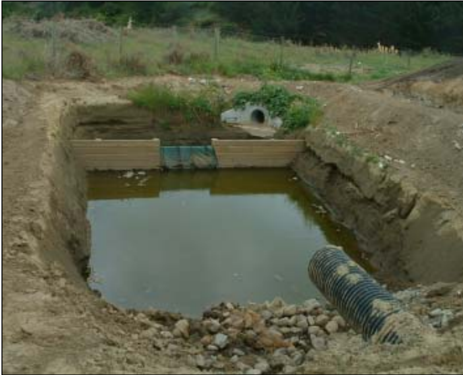
Photograph 3 New redesigned final settling pond, 27 November 2008
