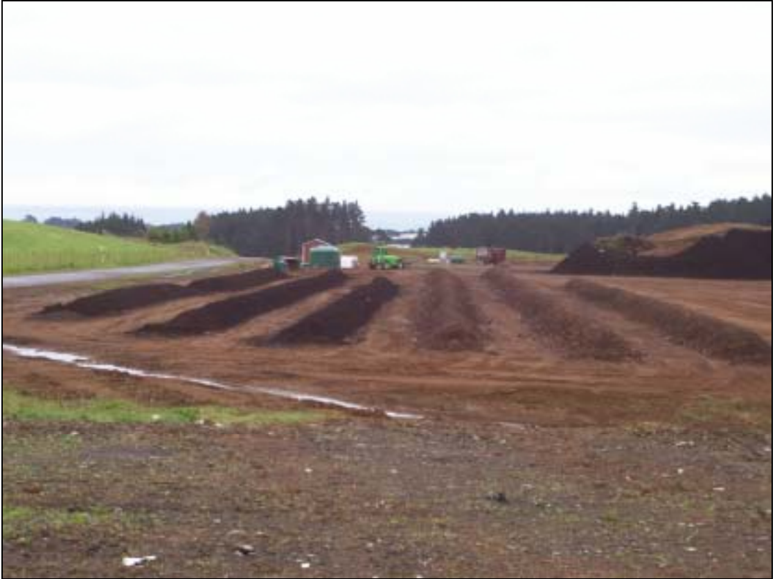
Photograph 2 Compost windrows at Colson Rd landfill, 28 October 2008
