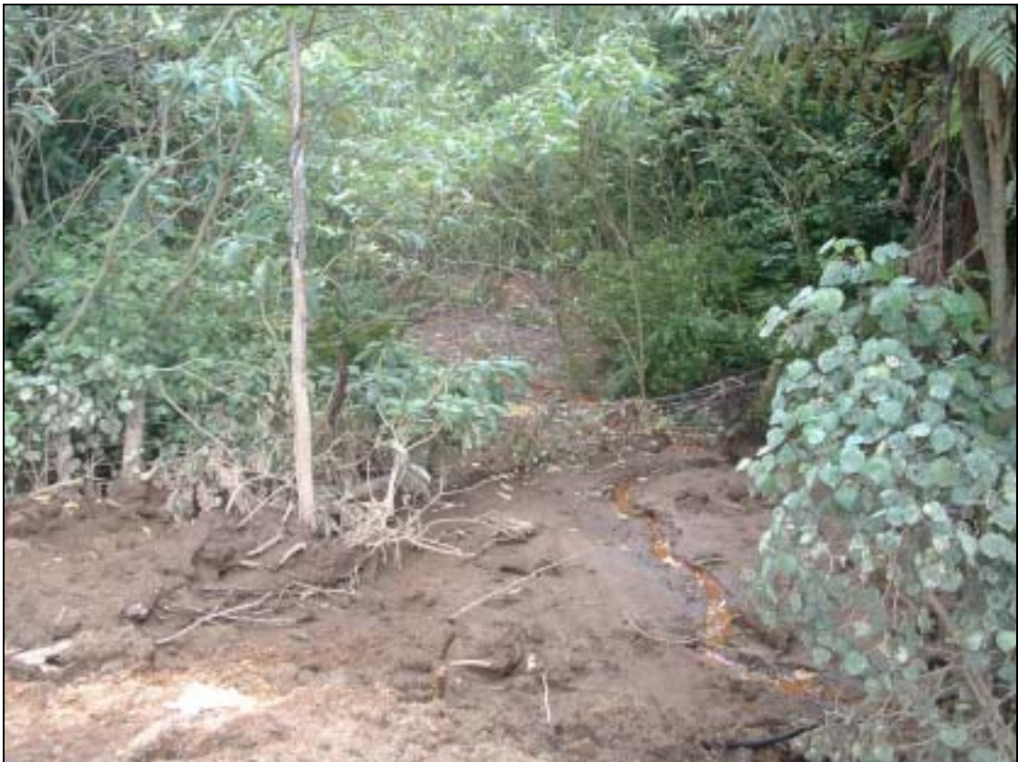
Photograph 6 Discharged silt from the small silt pond, 5 March 2009
