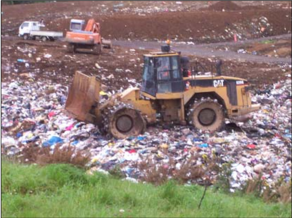
Photograph 4 Thirty six tonne rubbish compactor in operation, 28 October 2008
