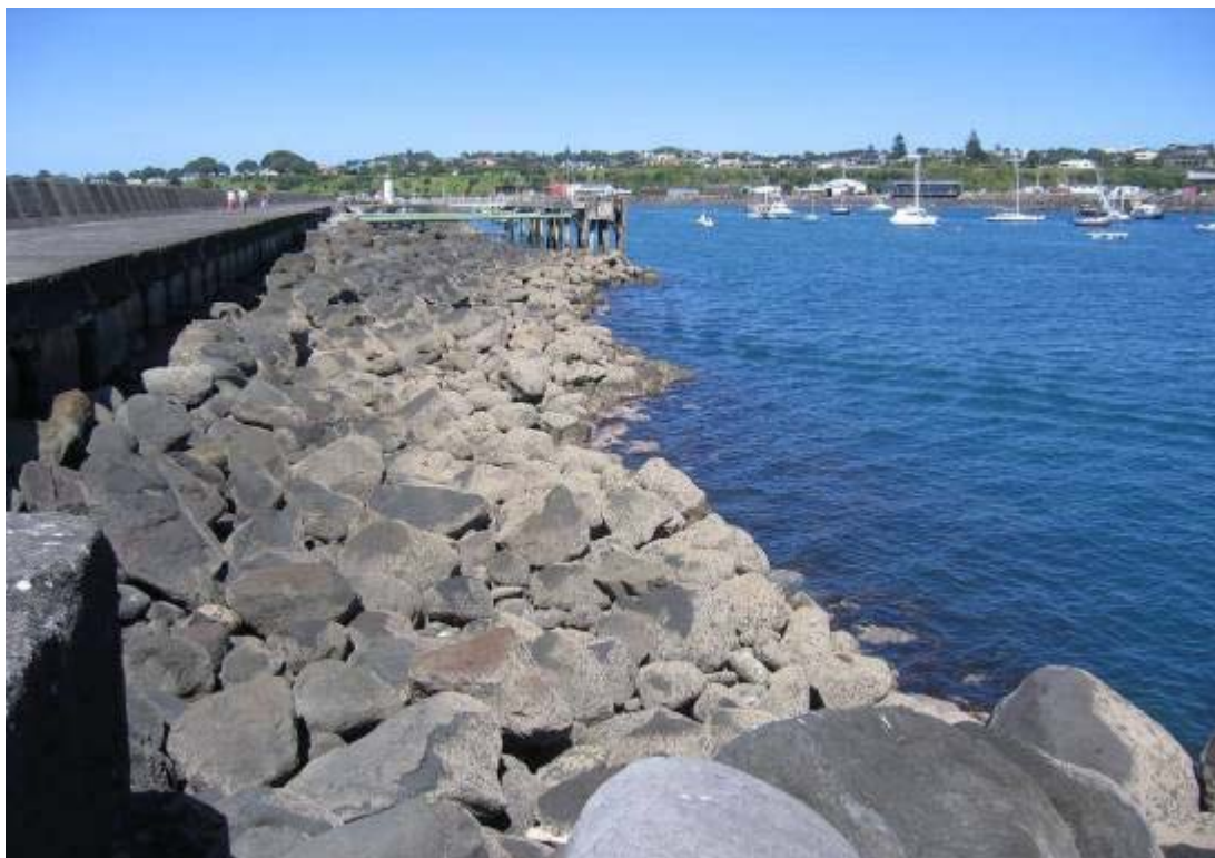
Photograph 3 Site inside the Lee Breakwater
