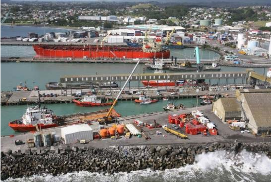
Photograph 1 Port Taranaki with the Main Breakwater in the foreground and Moturoa Wharf behind. The large ship is docked at the Newton-King Tanker Terminal while containers are visible on Blyde Wharf in the background
