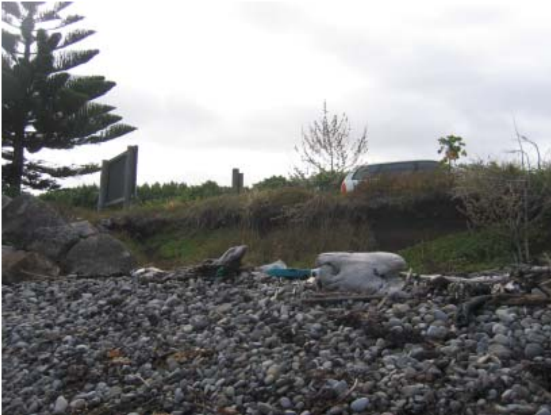
Photograph 9 Erosion at the end of the Bayly Road seawall, Cape Egmont
