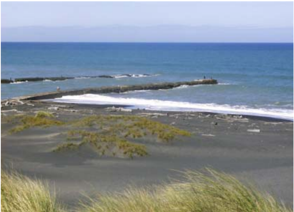
Photograph 5 Patea River groynes
