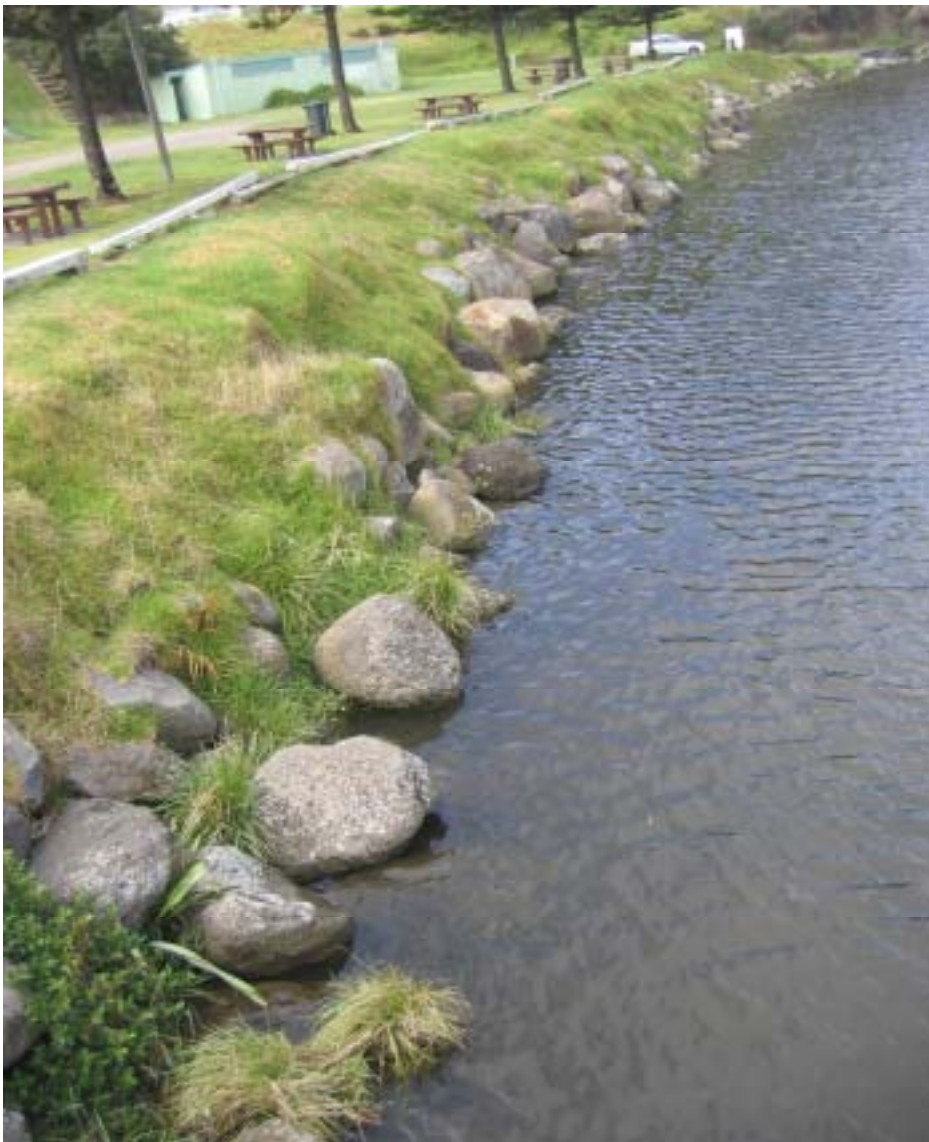
Photograph 3 Looking upstream along rock protection works in the Kaupokonui Stream
