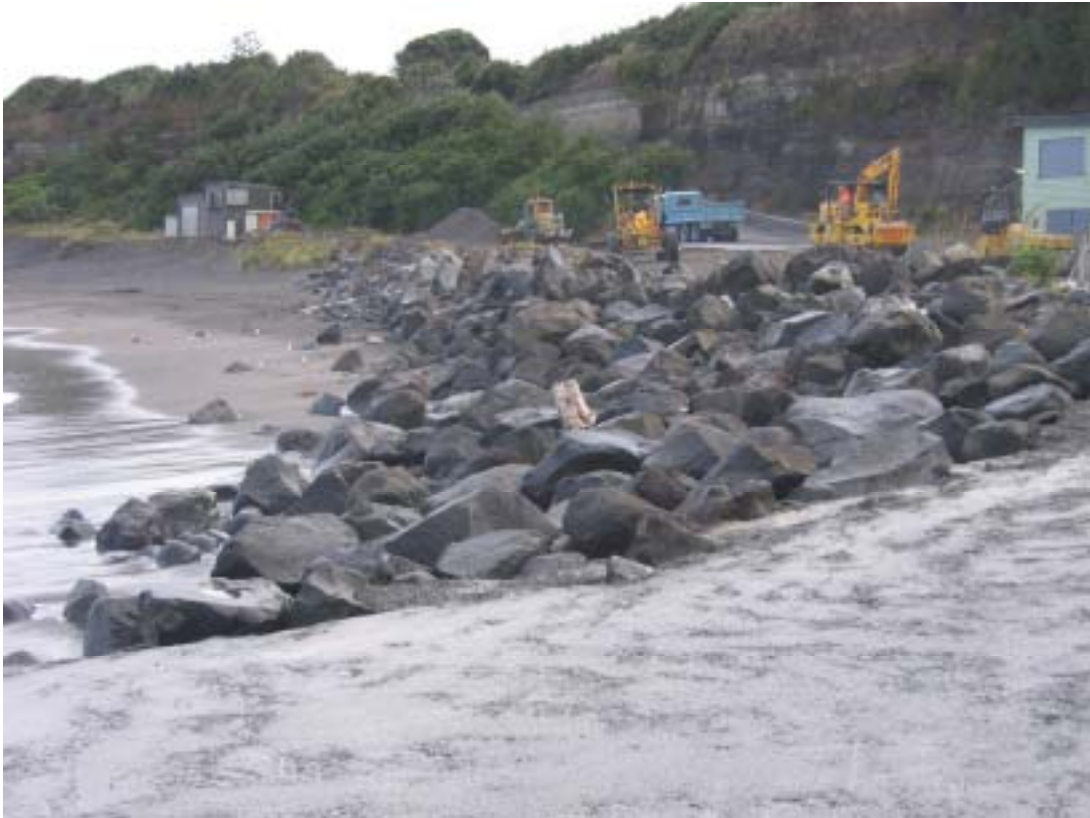
Photograph 10 Middleton Bay seawall
