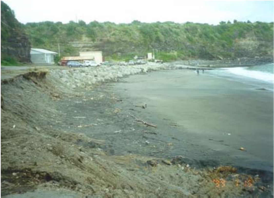
Photograph 1 Construction of rip rap seawall, Middleton Bay July 1999
