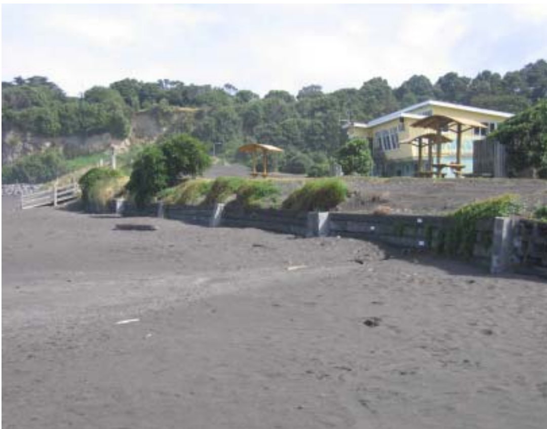
Photograph 2 A section of the Opunake Beach retaining wall
