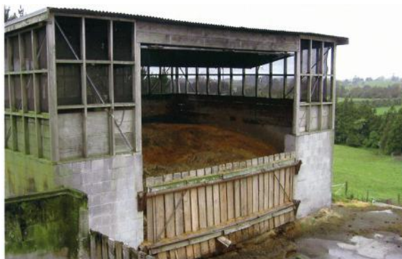
Photo 3 Covered aerated composting bunker
