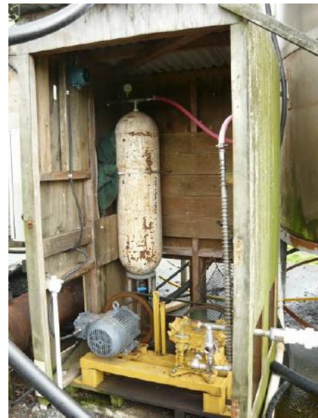
Photo 6 Biogas compressor
