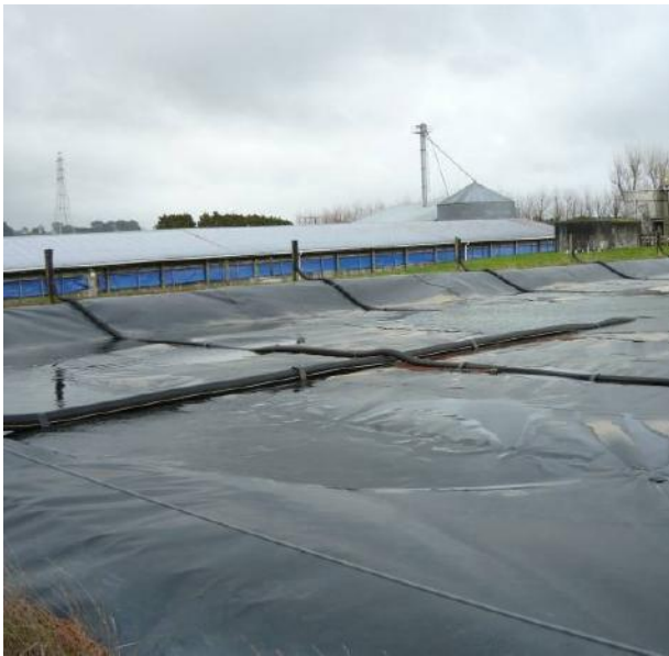
Photo 5 Covered anaerobic pond
