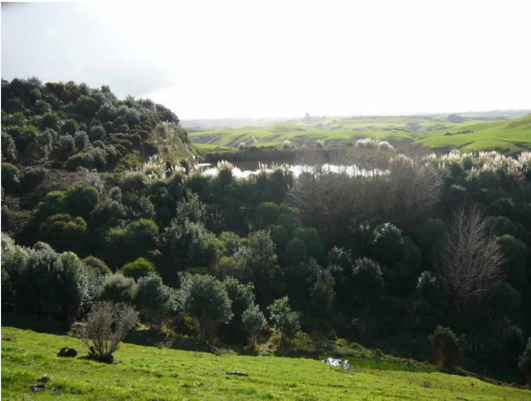
Photo 2 Looking north across the gully to oxidation pond treatment system
