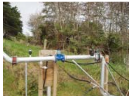
Good installation, sufficient straight length of pip between flowmeter and fittings and bends
