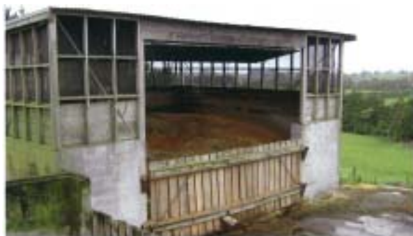
Photo 2 Covered aerated composting bunker
