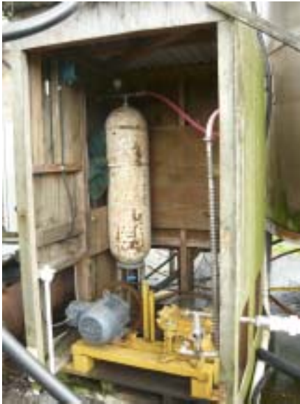
Photo 5 Biogas compressor
