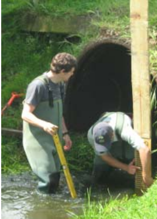
Photo 4 Installation of a staff gauge at a new control point
