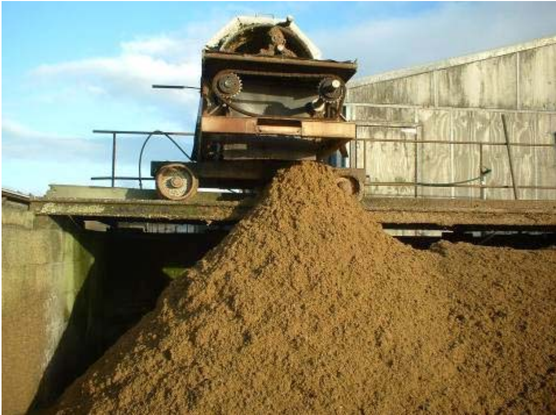
Photo 1 Solids separation and collection system
