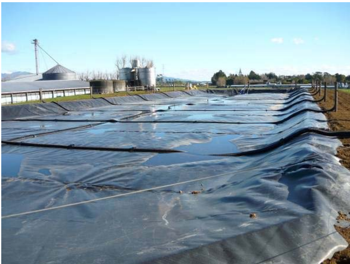
Photo 3 Covered anaerobic pond – flexible drainage pipes holds the covered in situ and protects the cover from severe wind
