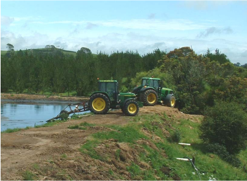
Photo 1 Sludge removal from second anaerobic pond
