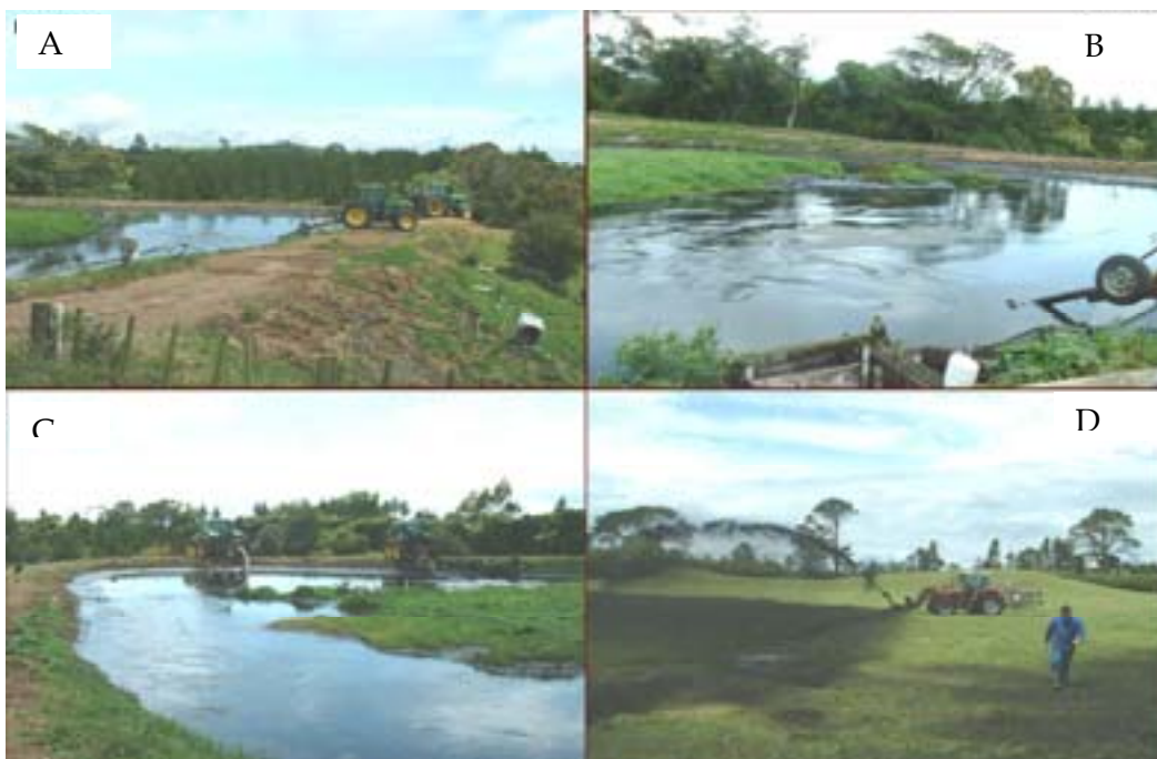
Photo 3 Sludge removal from second anaerobic pond (photos A to D)
