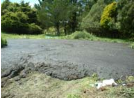
Photo 2 Drying sludge removed from the anaerobic pond
