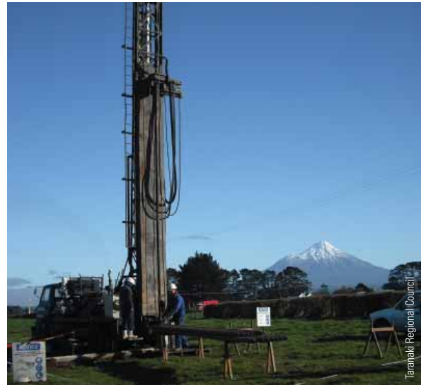
Drilling a water bore, Eltham.
