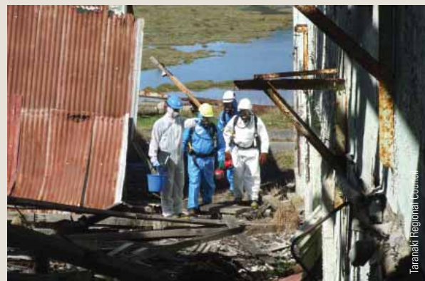
Taranaki Regional Council staff prepare to move hazardous waste after the fire.
