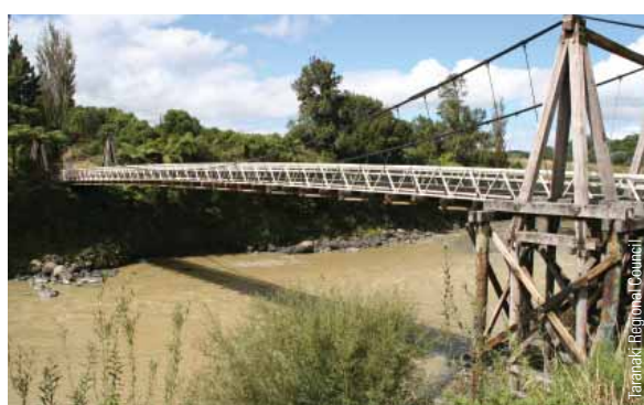
The historic wooden Bertrand Road Bridge over the Waitara River.
