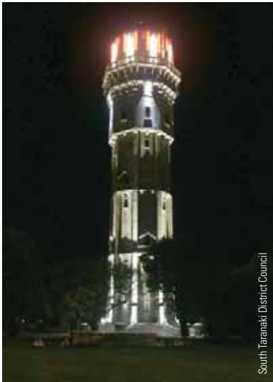
Hāwera water tower.
