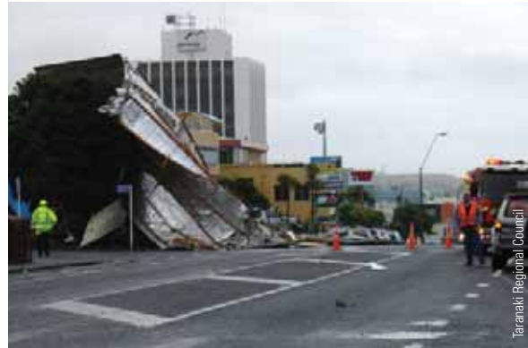
The roof from Placemakers landed across the street after the 4 July tornado.
