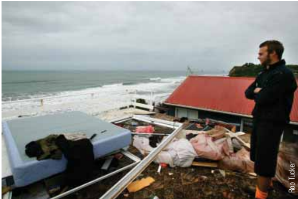
A resident surveys damage from the 5 July tornado, Ōākura.
