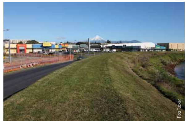
Flood protection works on the lower Waiwhakahiho River.
