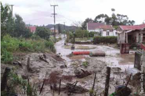
Flood damage, Waitōtara Township, 2004.
