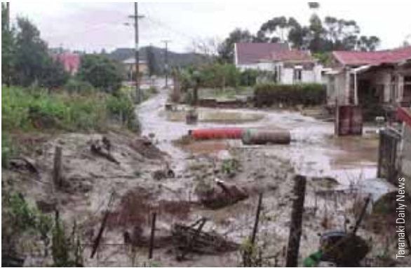
Flood damage, Waitōtara township, 2004.
