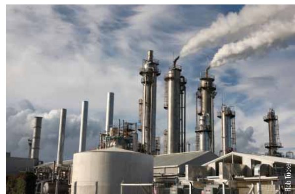
The Vector Kāpuni gas treatment plant.
