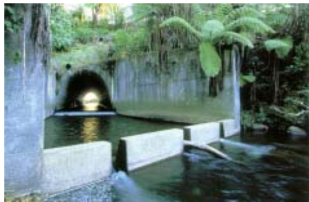
Through the consents process, modifications of this culvert on the Te Henui Stream involving the fitting of a fish pass ramp and wooden wedges to the floor have greatly enhanced fish passage
