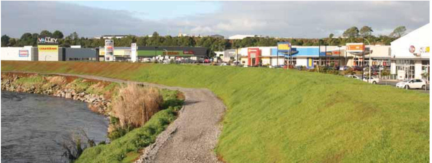
The raised stopbanks along Rifle Range Road.
