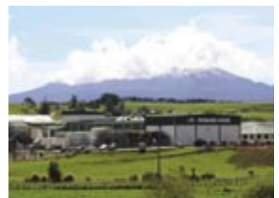
Riverlands Eltham Limited established its own wastewater disposal system to enable the company to expand.
